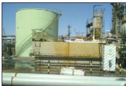
Basin in petrochemical complex.
