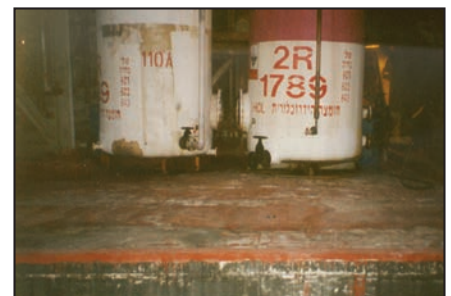
ARC 988 coated floor areas.
