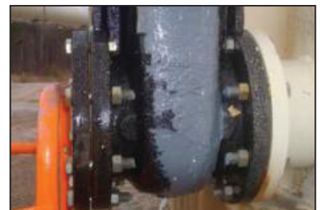
Repaired valve with ARC 5.
