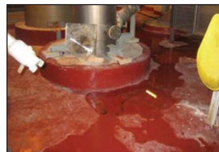
ARC NVE VC in service.
