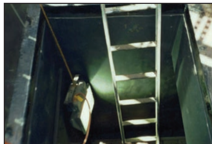
ARC specified by plant engineer.
