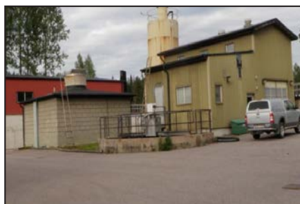
Wet well location.
