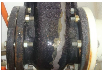
Valve leakage plugged with ARC 5ES.
