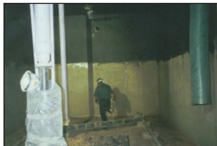
Concrete protected with ARC 791 and ARC 988 .
