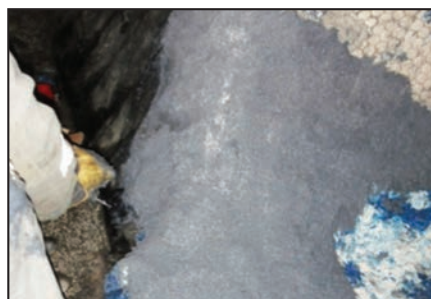
Applying ARC I BX1.
