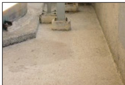
Cleaned and prepared surface.
