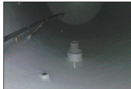
Coated tank internals.
