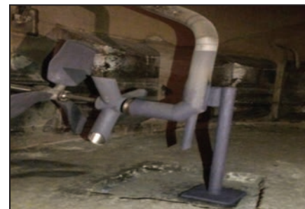
Design was modified to include additional support for the mixer and lance.
