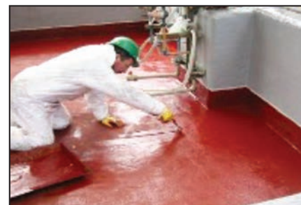
Applying ARC CS4 topcoat.
