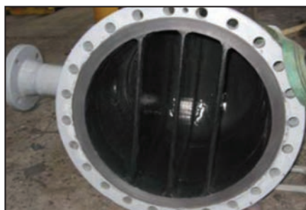
Repaired divider plates.
