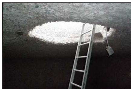
Surface of wet well high pressure cleaned and abrasive sweep sandblasted.
