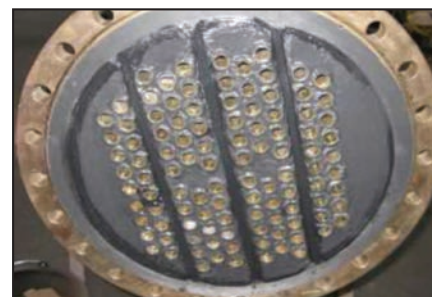
Completed tube sheet.
