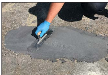
ARC EG-1 applied to concrete.
